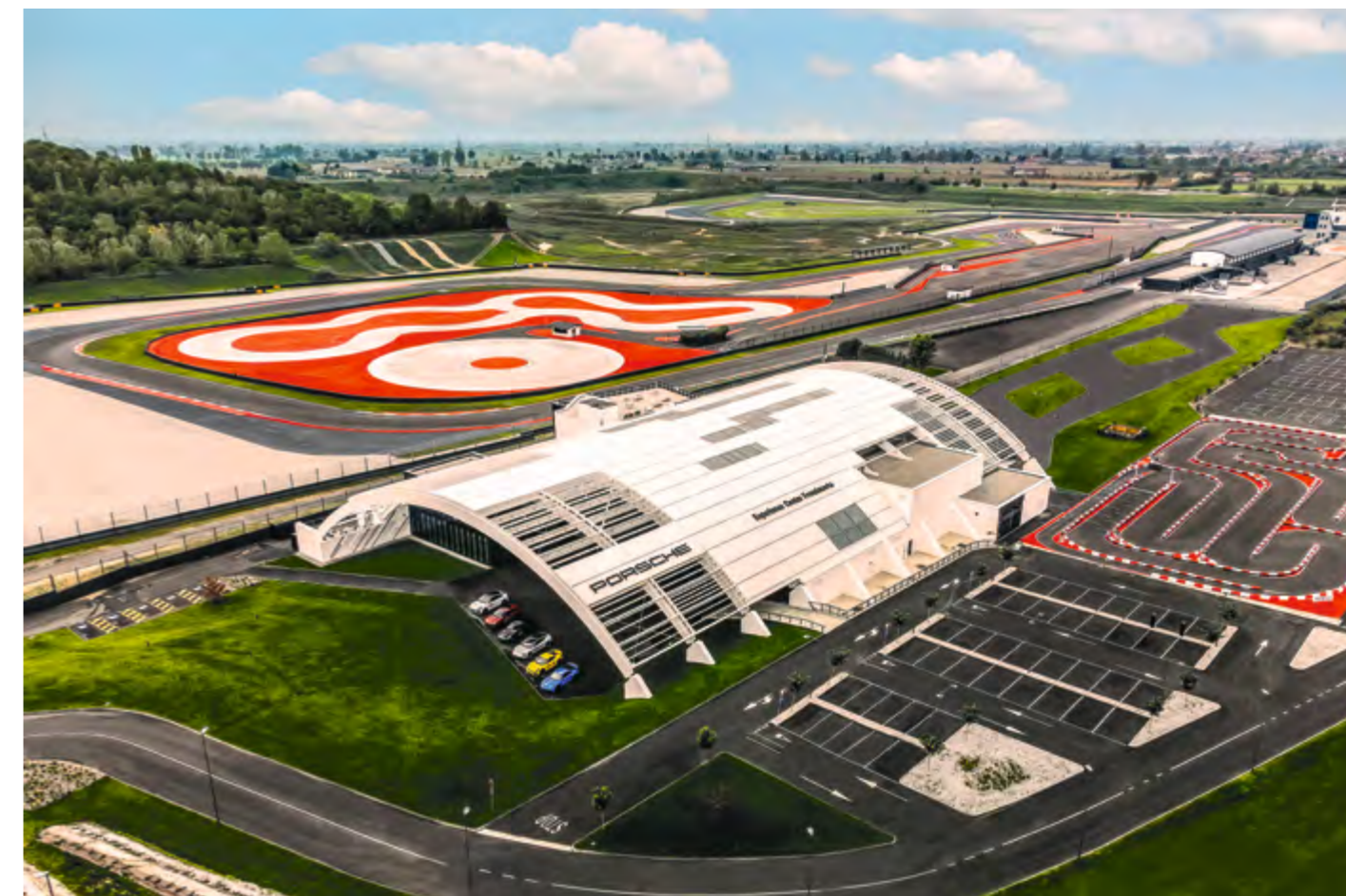
AERIAL VIEW OF THE NEW PORSCHE EXPERIENCE CENTRE IN FRANCIACORTA, ITALY
