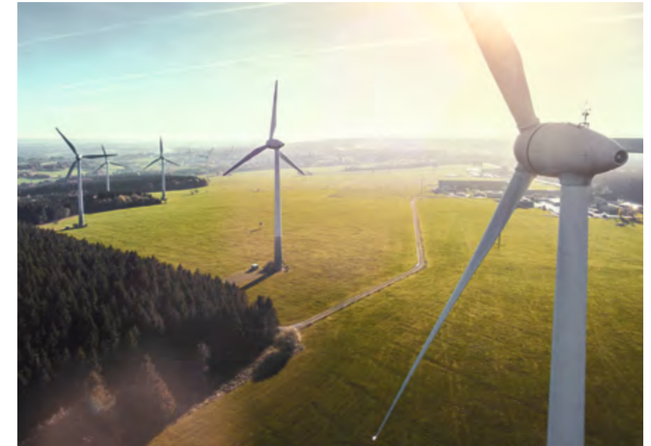
TRANSITION TO GREEN ELECTRICITY SUCH AS WIND POWER
